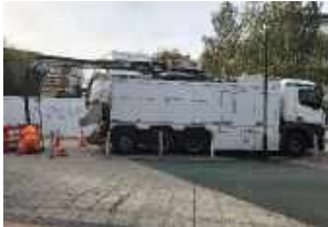
HIGH PRESSURE JETTING
